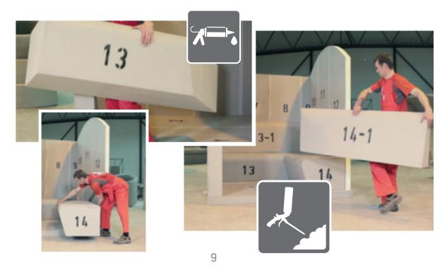
12. Once the benches have been set, it is time for corner board no. 15, which is again foamed and fastened using 3 thick blue screws!
