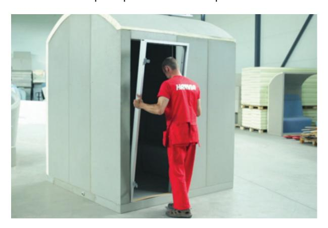
20. The door frame is first fastened from the top using a special screw. After this adjust the frame using a spirit level!
