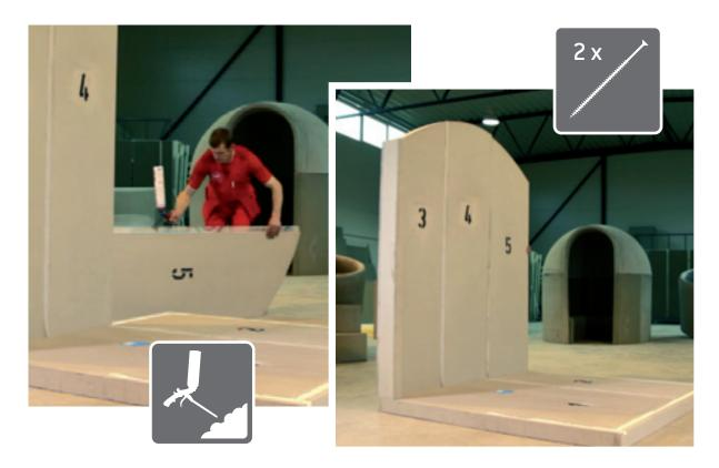
7. Element no. 6 is a corner board fasten it to the side of element no. 5 using 3 thick blue screws!
