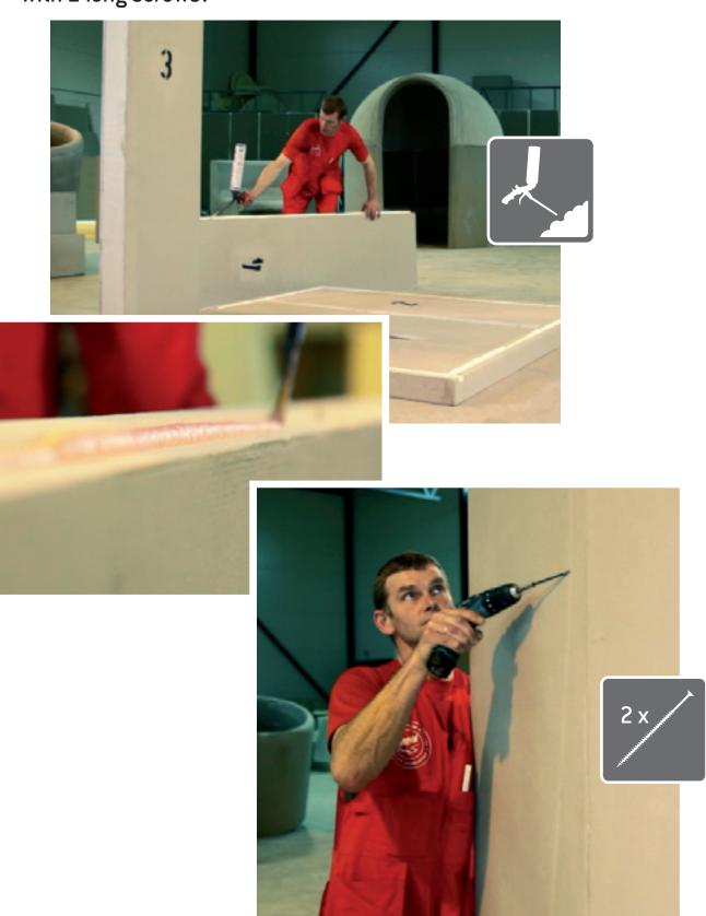
6. Repeat the same process with element no. 5 using foam and 2 long screws.
