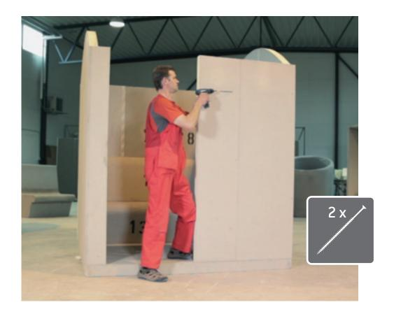
14. We've now reached the ceiling level, so let's start with element no. 18, which needs to be foamed first and then fastened using 3-5 longer screws as shown in the video!
