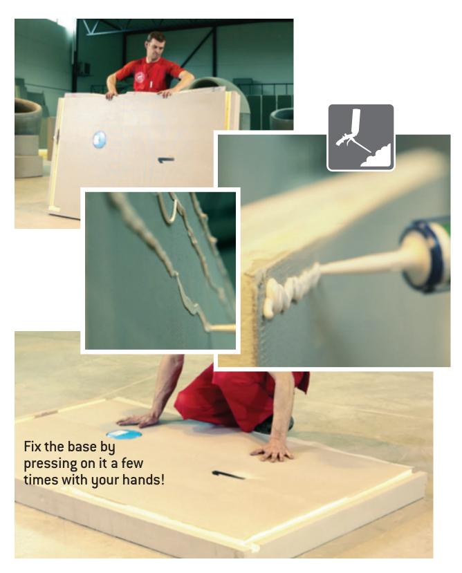
2. Next, take the element nr 2, apply glue to its bottom side just as with the first one, place it and fix by applying pressure with your hands.
