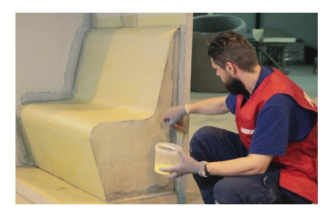
2. The first step in waterproofing is always the sealing of corners. Do this by applying wet membrane in the corners and gluing on the sealing tape. Next, cover the tape with the membrane as well.
