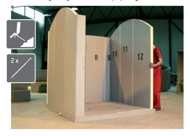
11. Installing steam room benches no. 13 and 14 is quick and easy as is the placing of backrests. Benches are fastened to backrests using glue or foam.
