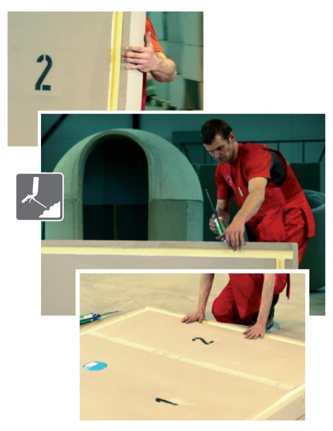
3. Use the glue gun to apply glue to the base grooves in full.
