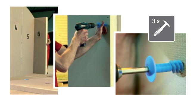
8. Remember to use the foam gun and the longer screws with elements 7, 8, and 9 to ensure a firm hold.
