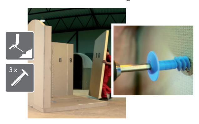
10. Fastening side walls 11 and 12 using foam and longer screws shouldn't cause you any sweat now. Keep up the good work!
