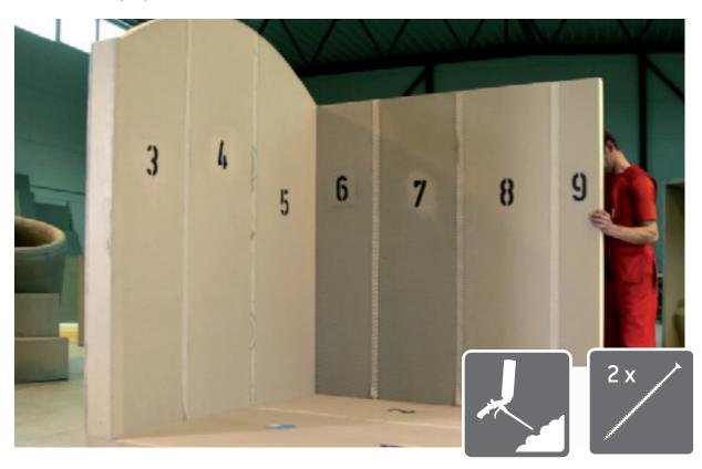
9. Element no. 10 is again a corner board that needs to be foamed and fastened into the side of element no. 9 using 3 thick blue screws.
