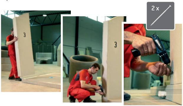
5. The side of element no. 4 needs to be covered using the foam gun before fitting it in the groove and then fastening the walls with 2 long screws!
