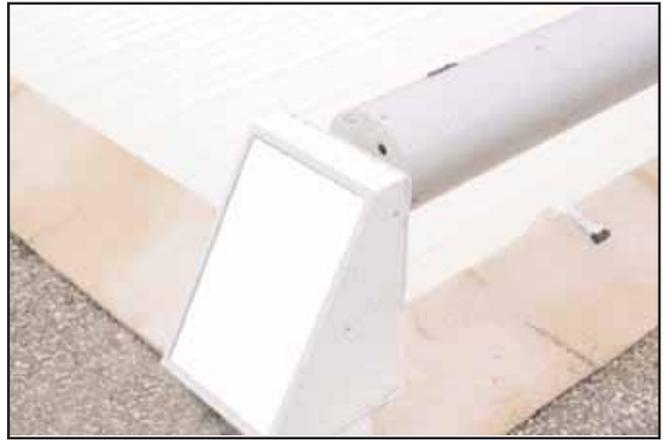
To finish, replace the casings on the stands and fix in position using the 4 screws M5-10.
