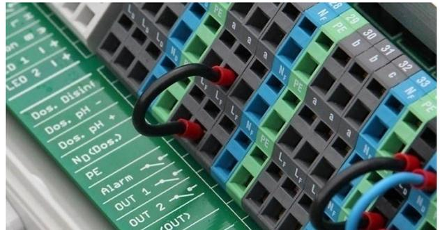
Wire bridge in the terminal box from phase L<sub>F</sub> to centre relay contact a
