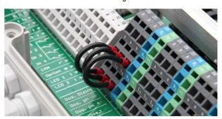
Wire bridges in the terminal box from phase  $L_{\text{\scriptsize D}}$  to the dosage outputs' centre relay contact a
